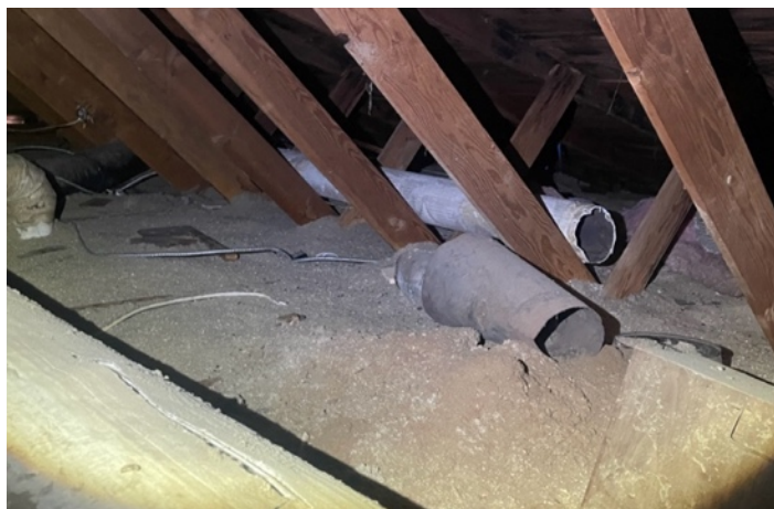
Example of the condition of a home attic before EASE Home upgrade includes fully disconnected ducts with asbestos and signs of rodent activity.
